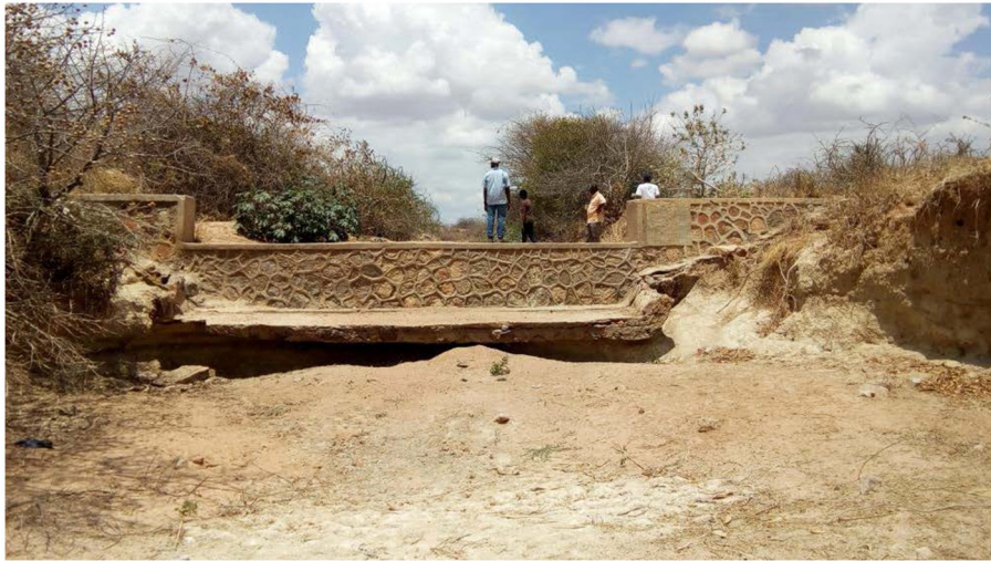
FIGURE 4 | Mshikamano sand dam near Dodoma, Tanzania exhibiting significant erosion of the apron and left streambank. Photograph taken while looking upstream during the dry season. Photo credit: J. A. Eisma.
