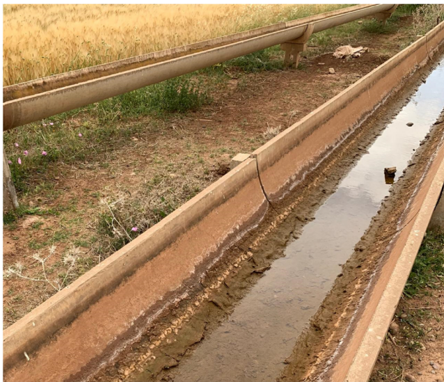
Fig. 2. Irrigation system consisting of elevated concrete canals arranged in a hierarchical structure.
