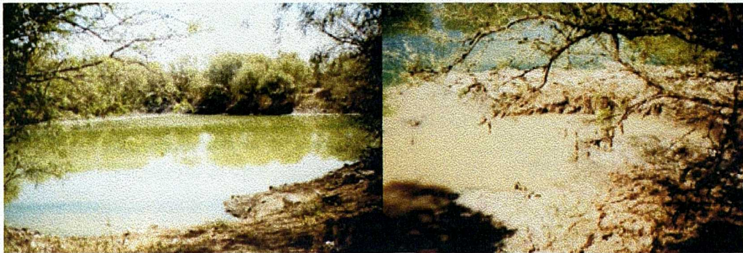
Figure 4.25. Sludge accumulation in the oxidation pond
