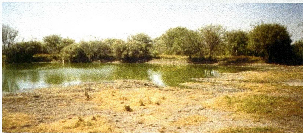
Figure 4.30. shows the basin (almost empty) used by one farmer to store the effluent of the pond until he decides to irrigate his parcel. Depending on the detention time, this basin can improve the quality of the effluent.
