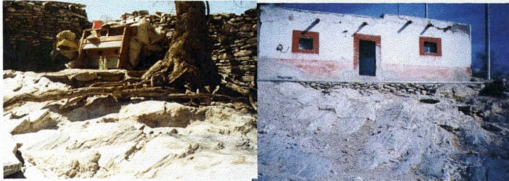
Figure 4.32. Houses built on the rock
