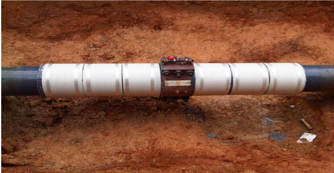
Figure 10. Crack repair using crack arrestors [163]
