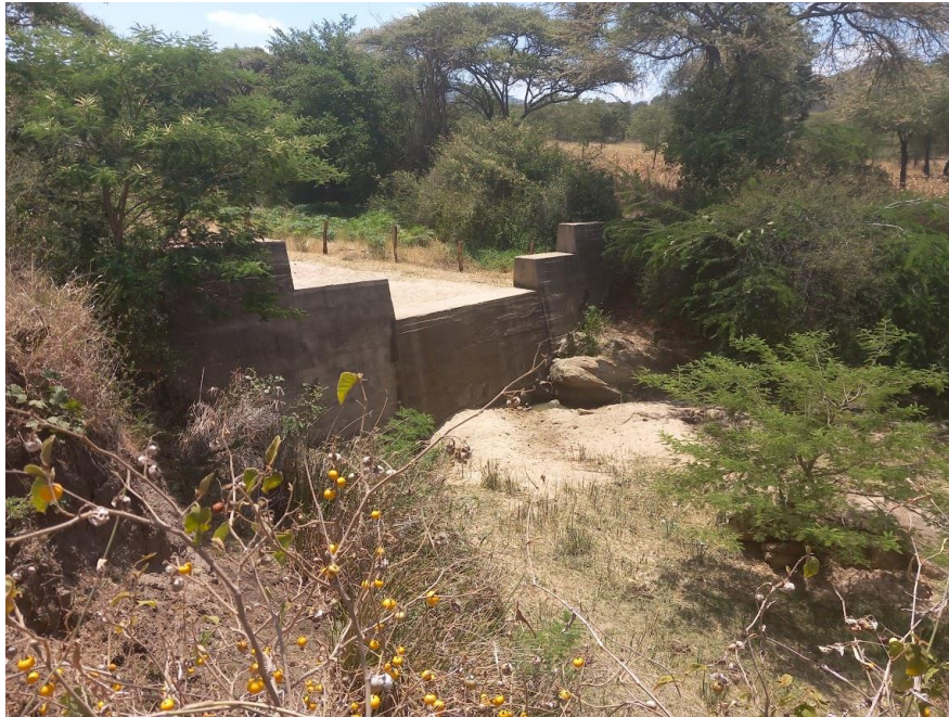
Figure 1-2: Sand dam in Makueni County, Kenya. Dam wall consists of central spillway, 2.8 m in height, and wingwalls. Together they measure 23 m in length here. Trapped alluvium accumulated behind the dam wall extends 245 m upstream here (Ritchie, 2023).
