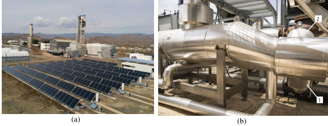
Fig. 3. HC pilot plant at PSA-CIEMAT: a) flat-plate collectors of the heating circuit, b) steam generator: hot water inlet (1) and outlet (2).
