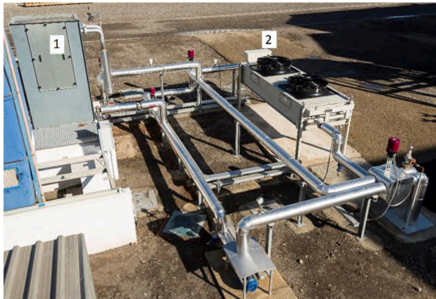
Fig. 5. Cooling circuit in the HC pilot plant at PSA-CIEMAT. WCT (1) and ACHE (2)
