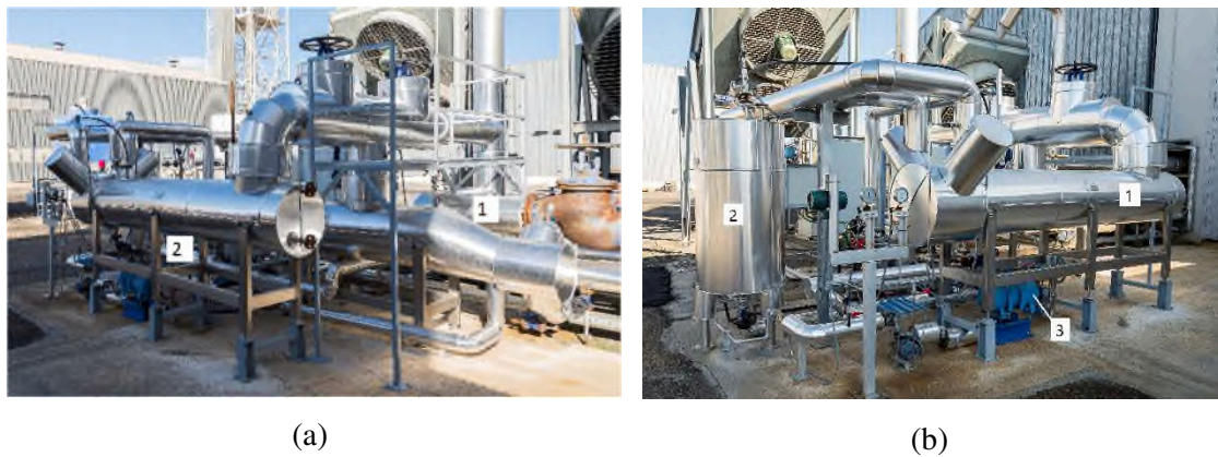
Fig. 4. HC pilot plant at PSA-CIEMAT, exchange circuit: (a) steam generator (1) and surface condenser (2), (b) surface condenser (1), condensate tank (2) and small deposit under the surface condenser (3).
