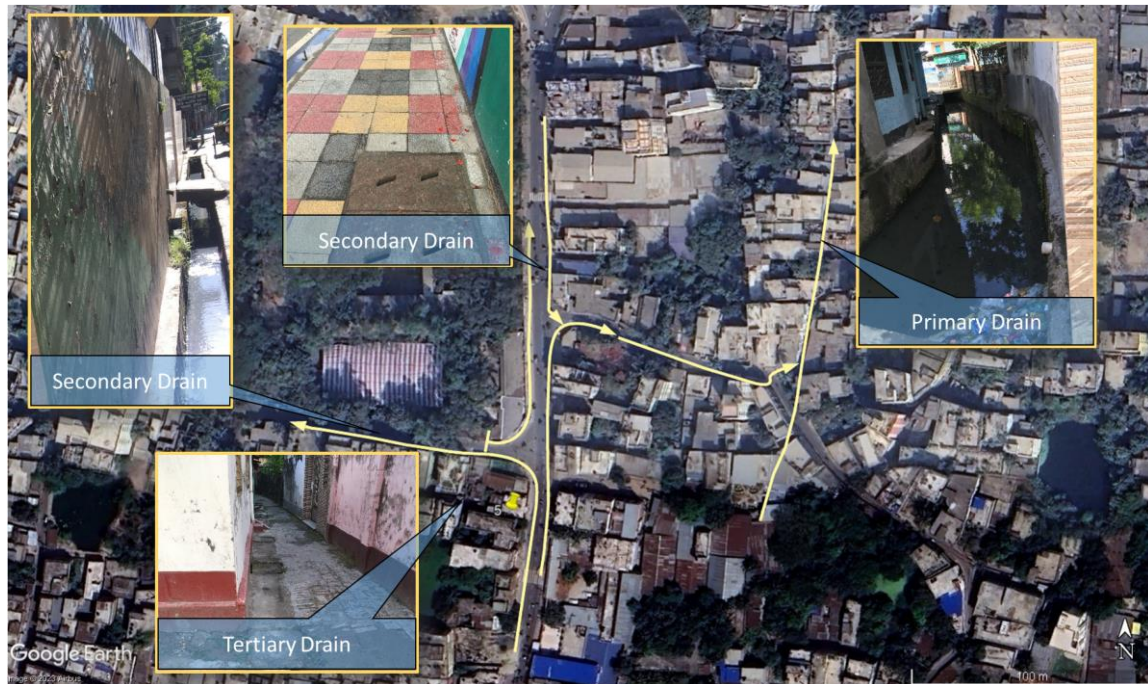
Figure 4.3: The primary drain has a width of more than 1 metre within the area which receives the flow from secondary drains (less than a metre in width) which in turn receive flow from tertiary drains of a width of less than half a metre.
