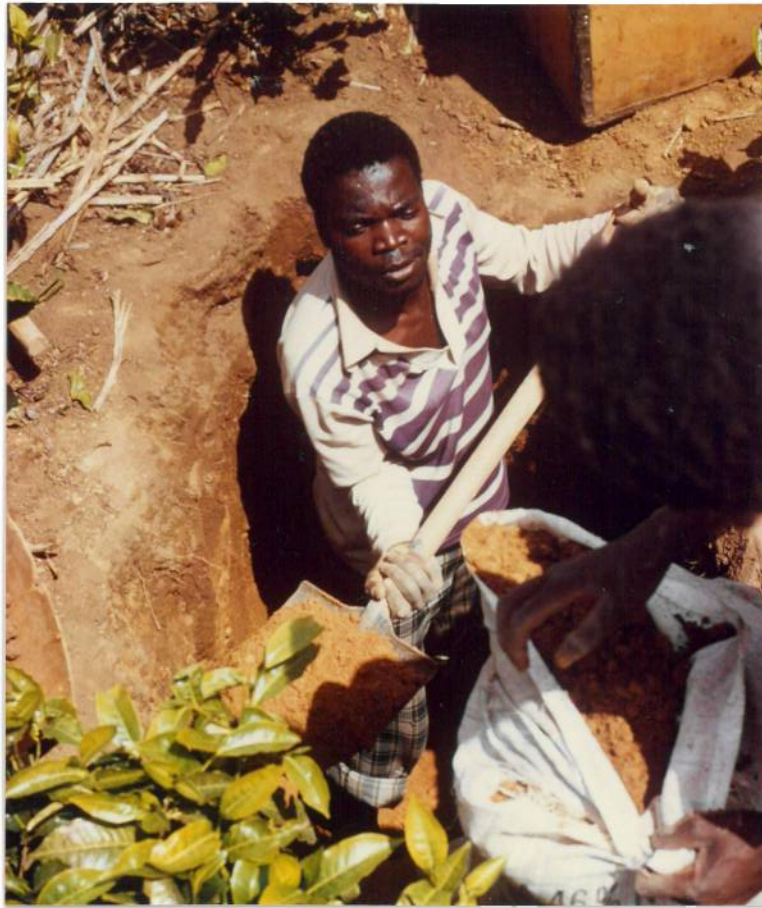
Plate 6.1. Excavation of roots
