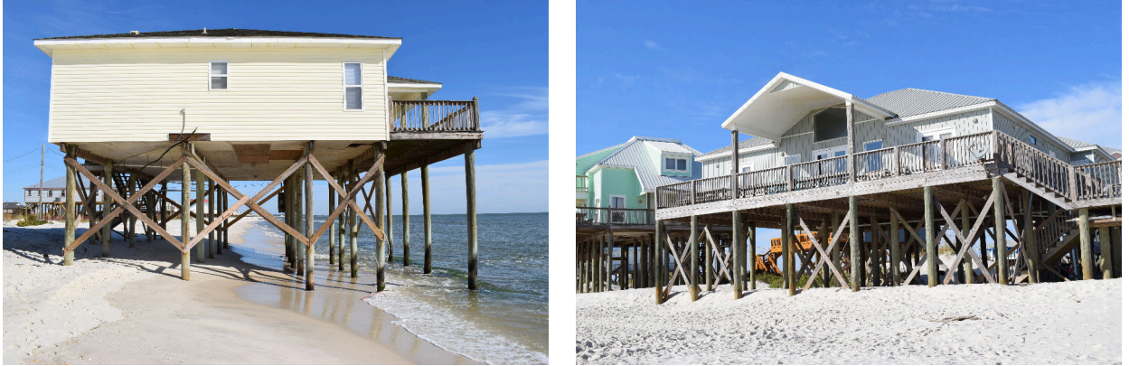
Figure 1: Photographs of elevated coastal residential houses on Dauphin Island, Alabama, USA. 27 Nov. 2016. Author's (Guoji Xu) personal collection.
