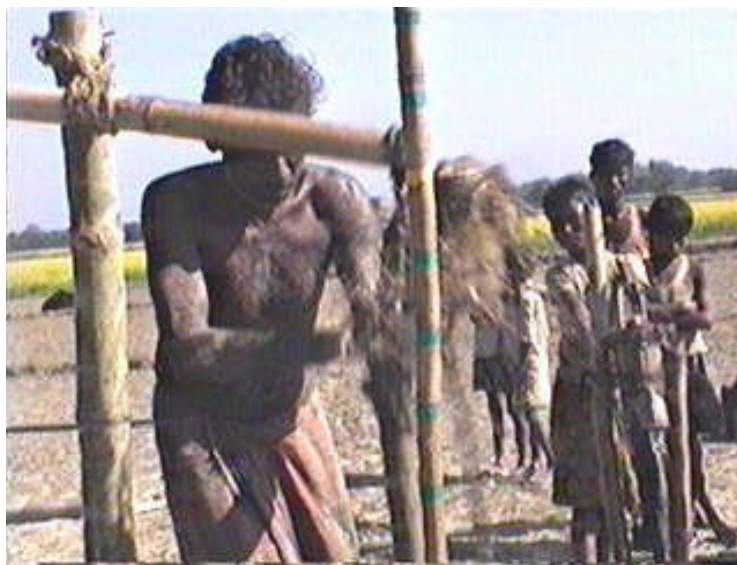
Figure 2: Sludge Ejecting from the Pipe
