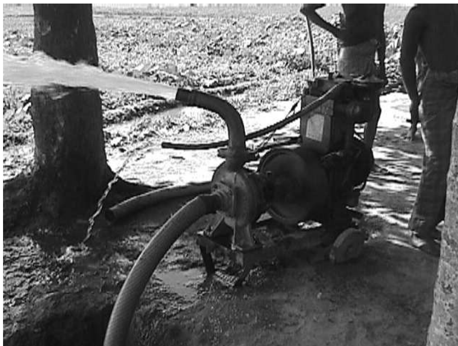
Figure 18: Flow from an Installed 3" Diesel Pump
