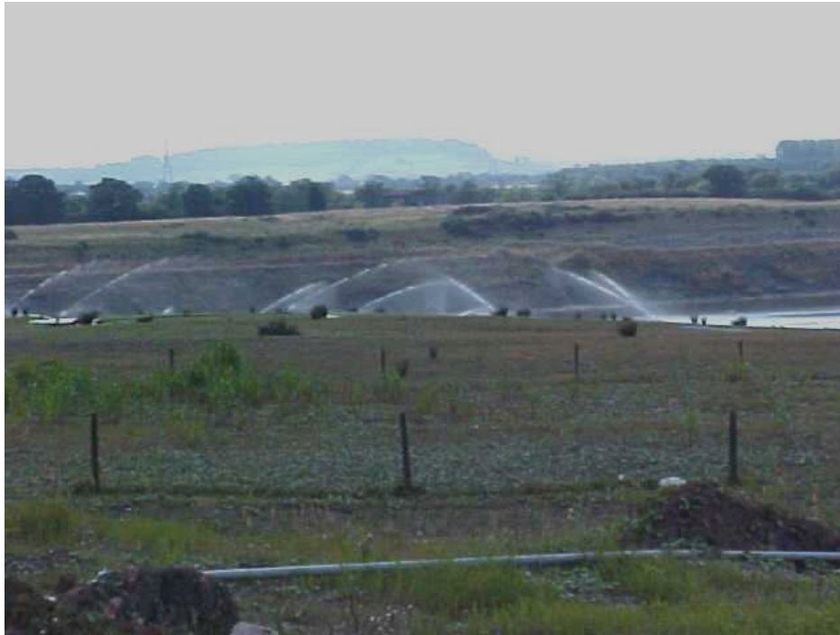
Fig. 1. Representative spray irrigation of landfill leachate using spray guns and illustrating typical spray radii
