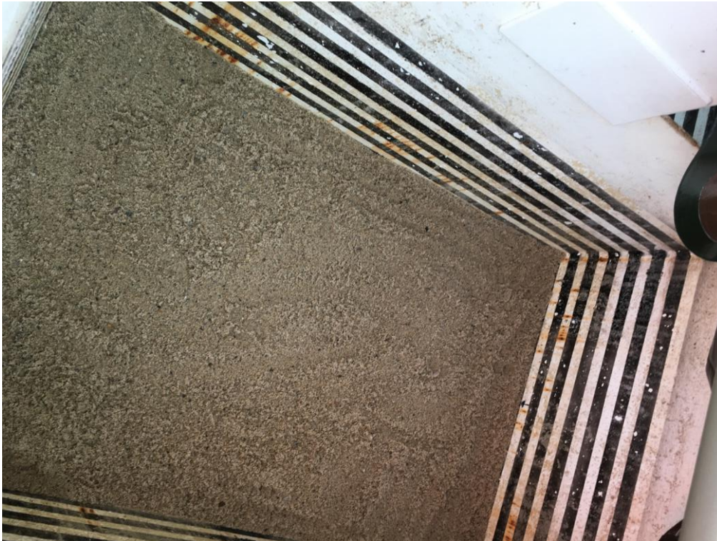
Figure 5.4: Image of one of the filters before operation, showing the 20 mm graduated lines used to guide skimming depth.
