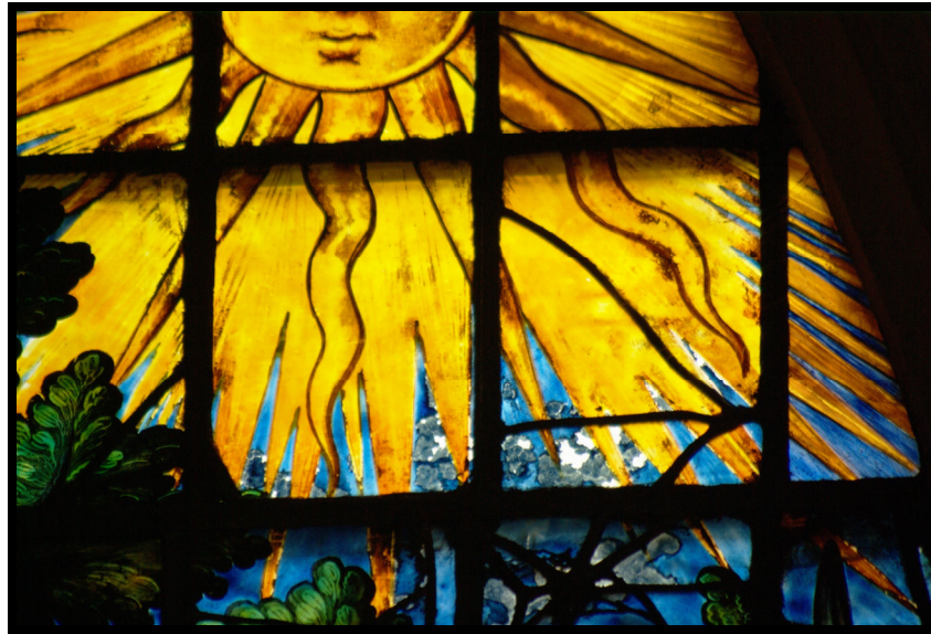
Figure 3-86 Left hand light showing the flaking paint
