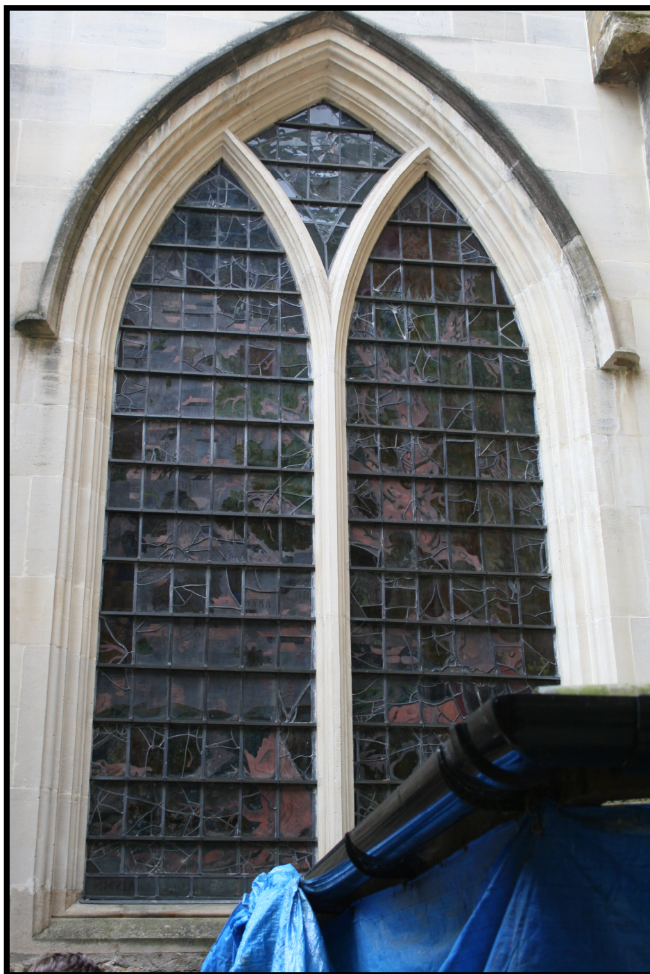
Figure 3-91 Photograph of the rear of the 'Jonah' window at Christ Church
