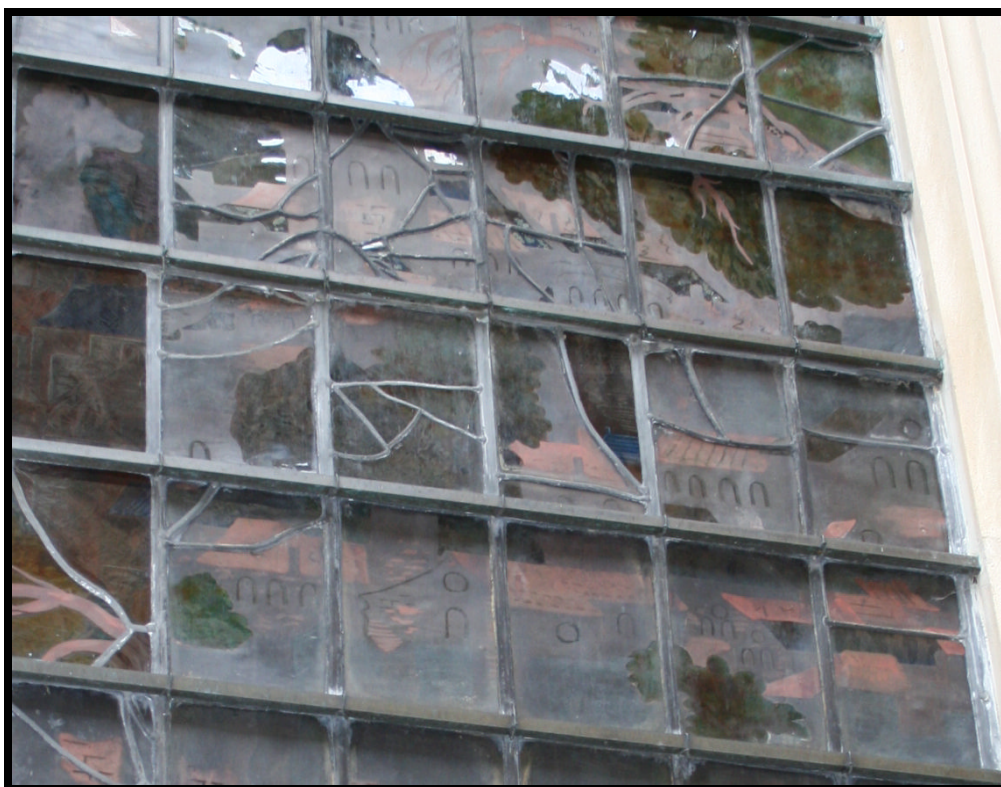
Figure 3-92 Close-up of the back-painted rear of the 'Jonah' window, on the left of the image can be seen a panel which is suspected to be a 'modern' restoration and the city is not back-painted
