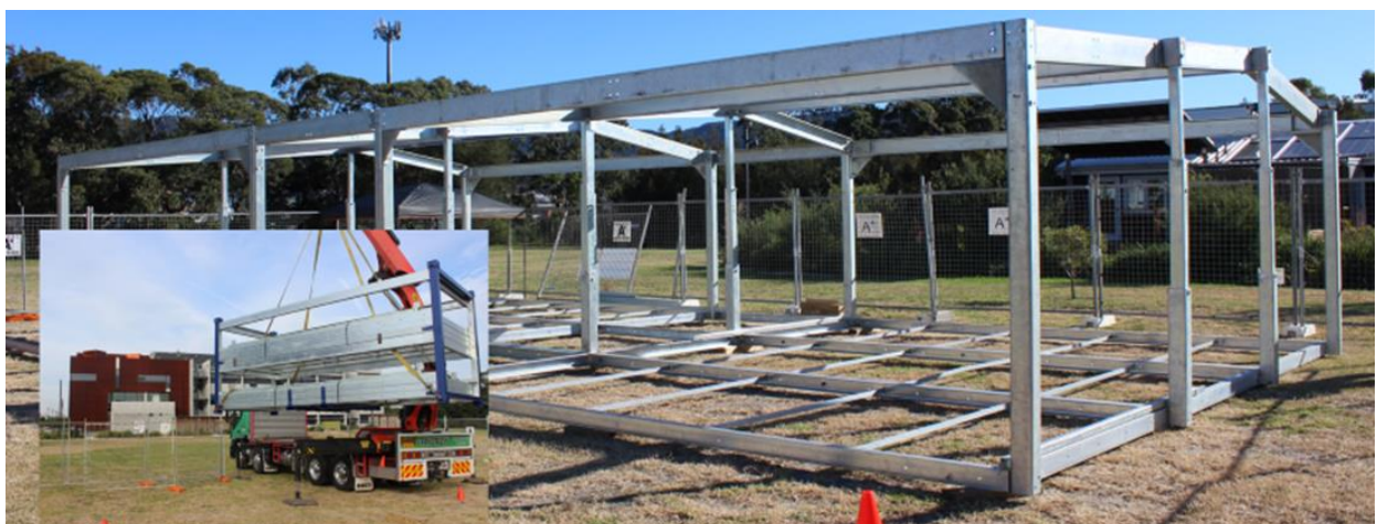
Figure 3: BuildCo's Structural Steel Housing System
