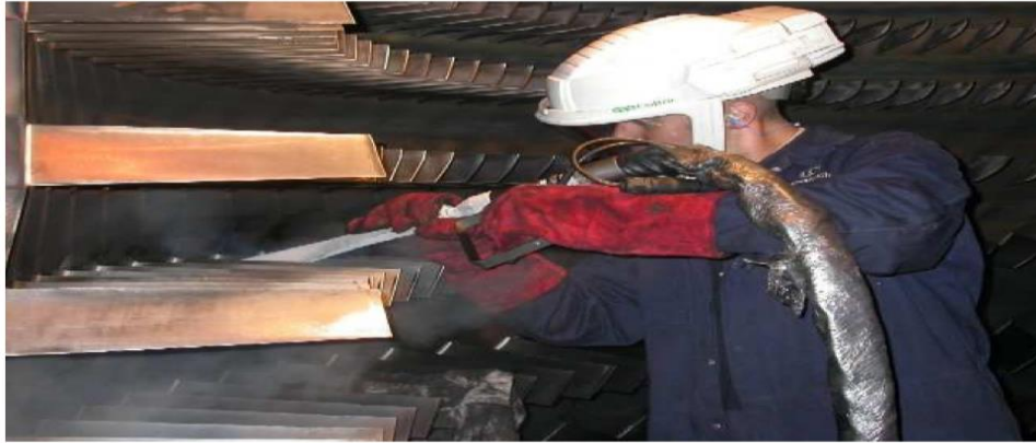
Figure 2-18 Manual cleaning of the compressor [113]
