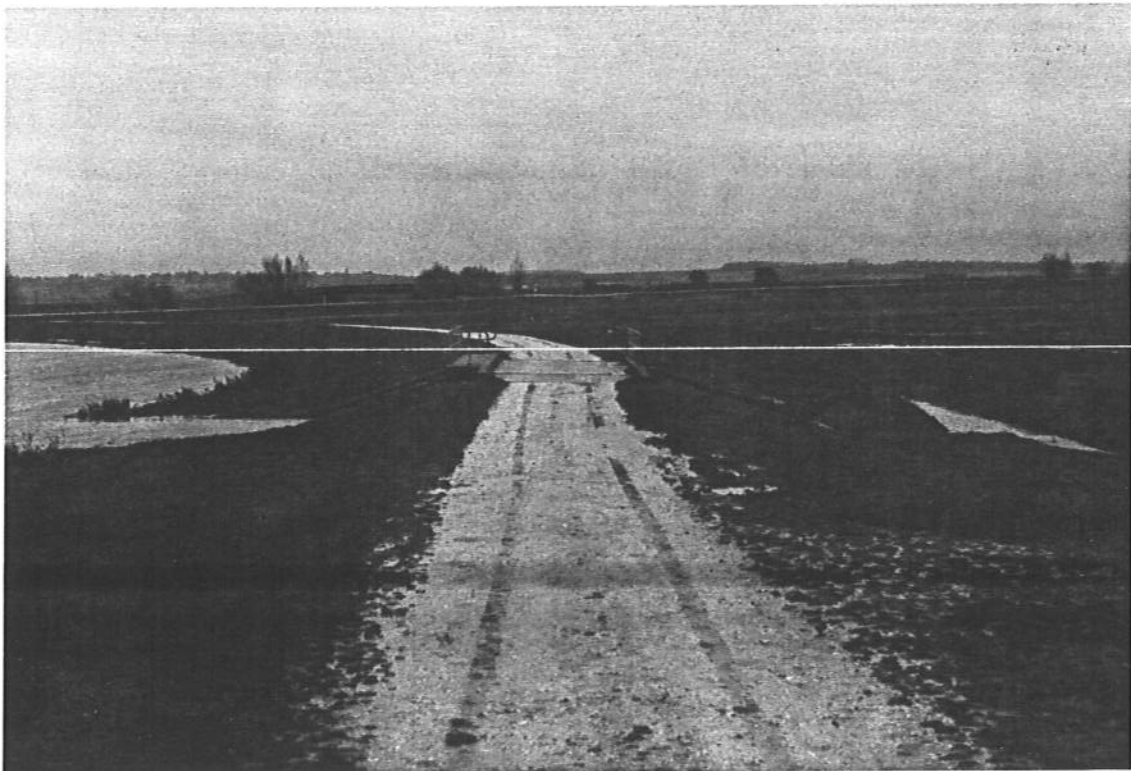
Plate 6: Outfall for Drains 38/40 near Idle Stop - December 1992
