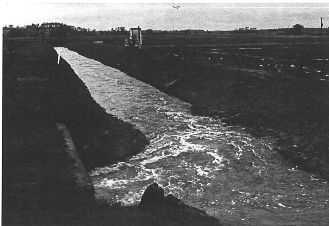
Plate 13: Wiseton Pumping Station in operation - December 1992
