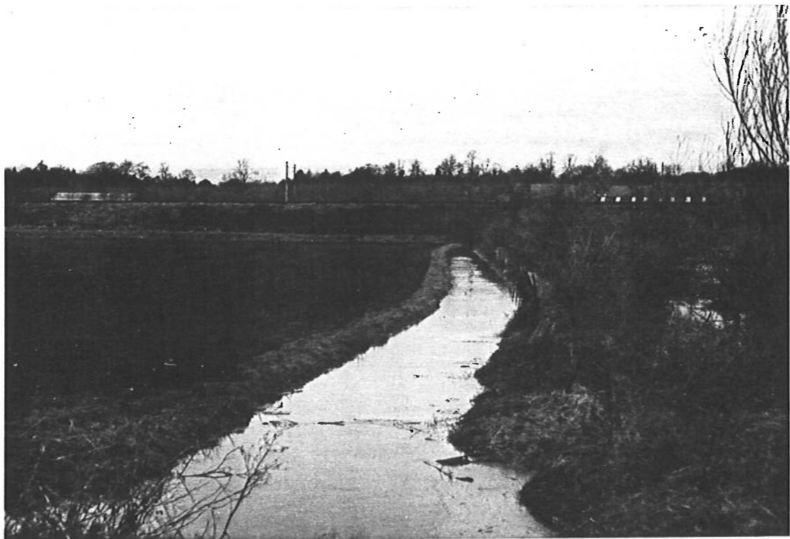
Plate 10: Drain 49 behind outfall at Bawtry Bridge - December 1992
