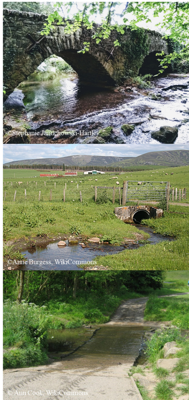
Figure 1. Examples of road–river infrastructure types (from top: bridge, culvert, ford) present in Great Britain. The ‘Culvert at Calier - geograph.org.uk - 1938882.jpg’ image has been obtained by the author(s) from the Wikimedia website where it was made available by Anne Burgess under a CC BY-SA 2.0 licence. It is included within this article on that basis. It is attributed to Anne Burgess. The ‘Ford though the River Lostock, Cuerdon Valley - geograph.org.uk - 1385002.jpg’ image has been obtained by the author(s) from the Wikimedia website where it was made available by Ann Cook under a CC BY-SA 2.0 licence. It is included within this article on that basis. It is attributed to Ann Cook.
