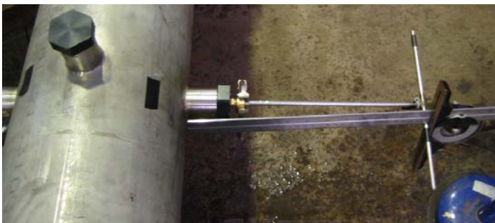
Figure 5.6: Beam pitot end installed through IPTS tapping points
