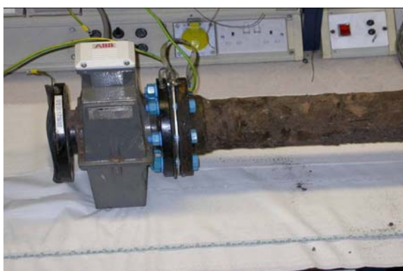
Figure 7.13: Meter condition - after removal of protective tape
