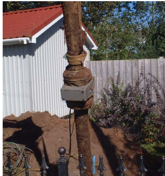
Figure 7.10: Removing SAM meter sensor 6891 from Manor Place
