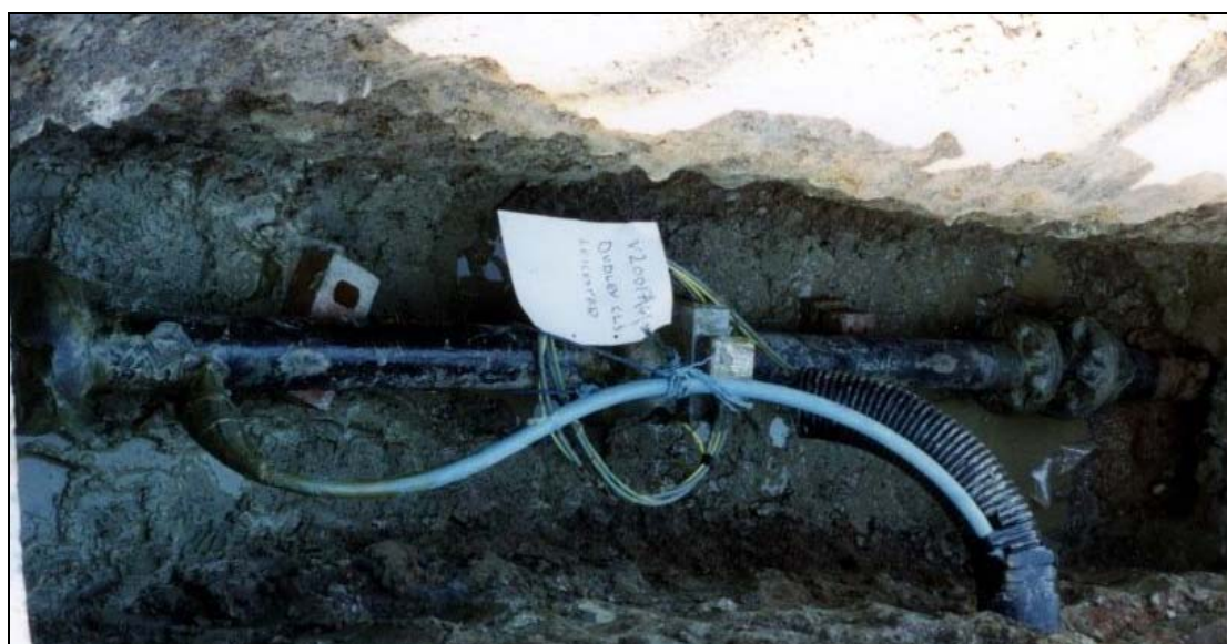
Figure 7.4: SAM Sensor installation in trench prior to burial
