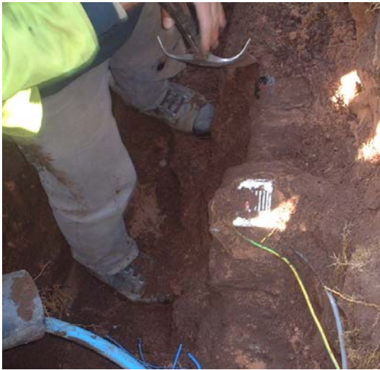
Figure 7.9: Excavating SAM meter sensor 6891
