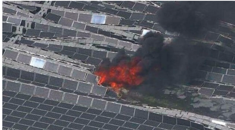
Figure 1. An accident of an FPV farm in Japan, subject to extreme wind conditions [24].
