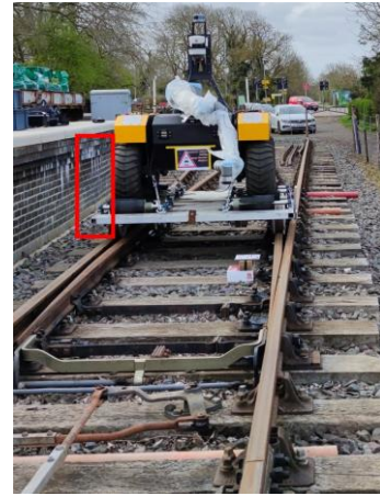
Fig. 4. Congested space between the track and platform
