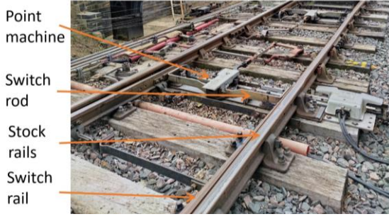
Fig. 5. Basic components of a switches and crossings
