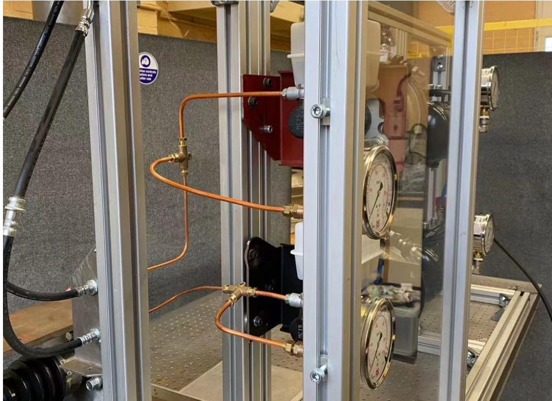
(e) The Final Copper Pipe Connection
