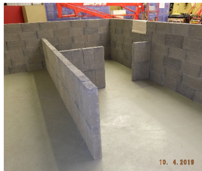
Figure 1 Concrete building structure
