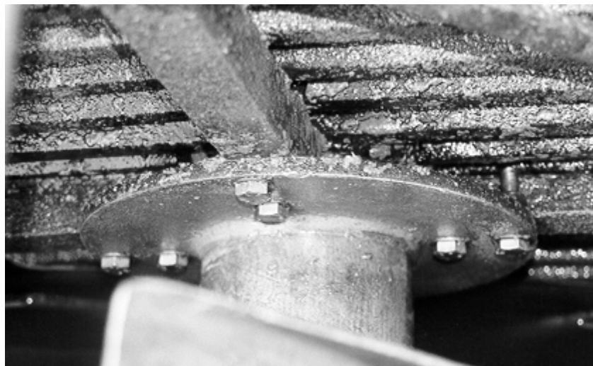
Figure 45 Welded shaft plate
