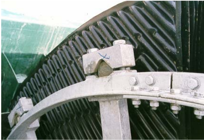
Figure 82 Four-point line contact ‘vee’ block
