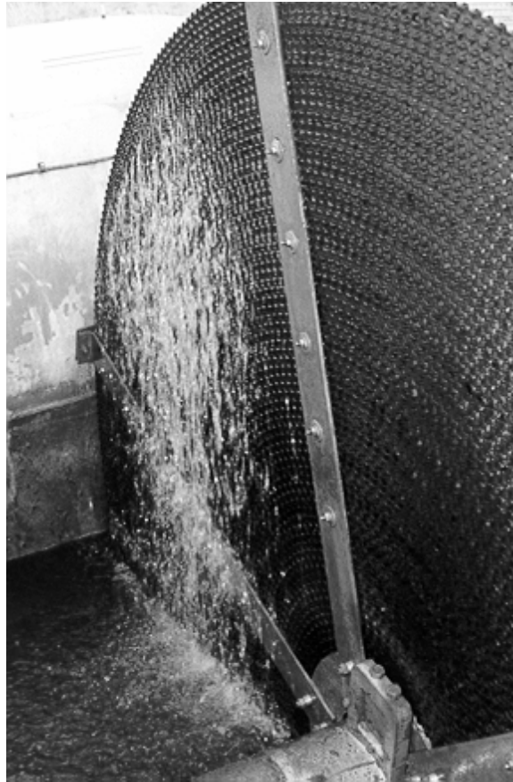
Figure 50 Support structure design arrangement for trapezium type media corrugations
