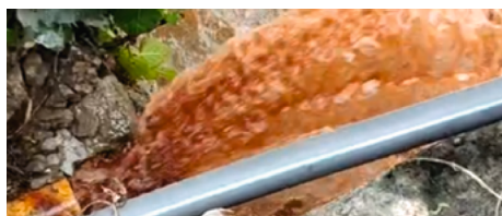
(a) On-site cleaning underground pipes
