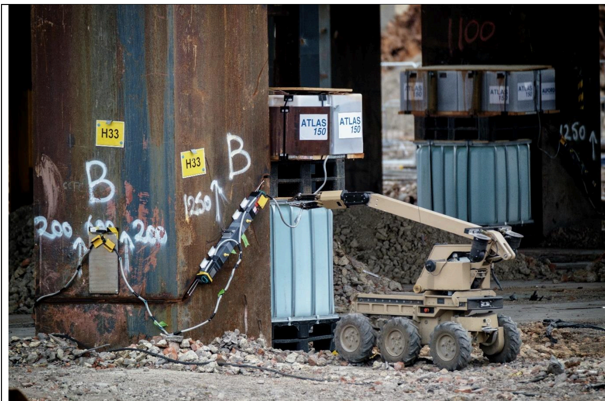
Fig 4. The modular ATLAS 150 was designed and developed specifically to kick columns out of alignment. The Magnetic Bunch Connector board can be seen with two protected detonating cord links.
