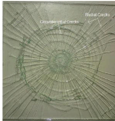
Figure 9. Radial and circumferential crack patterns in laminated glass.
