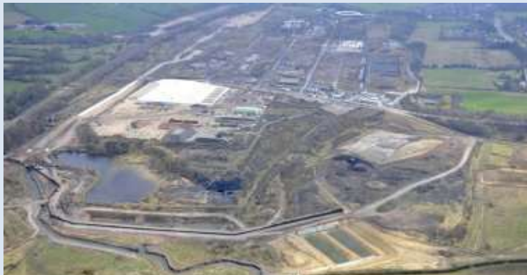
Aerial view of the site – during remediation
