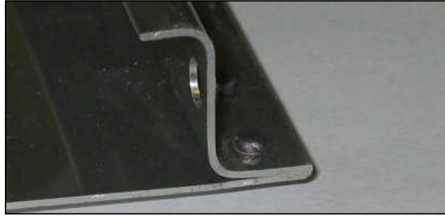
Figure 10: Curved Shape of a Stiffener
