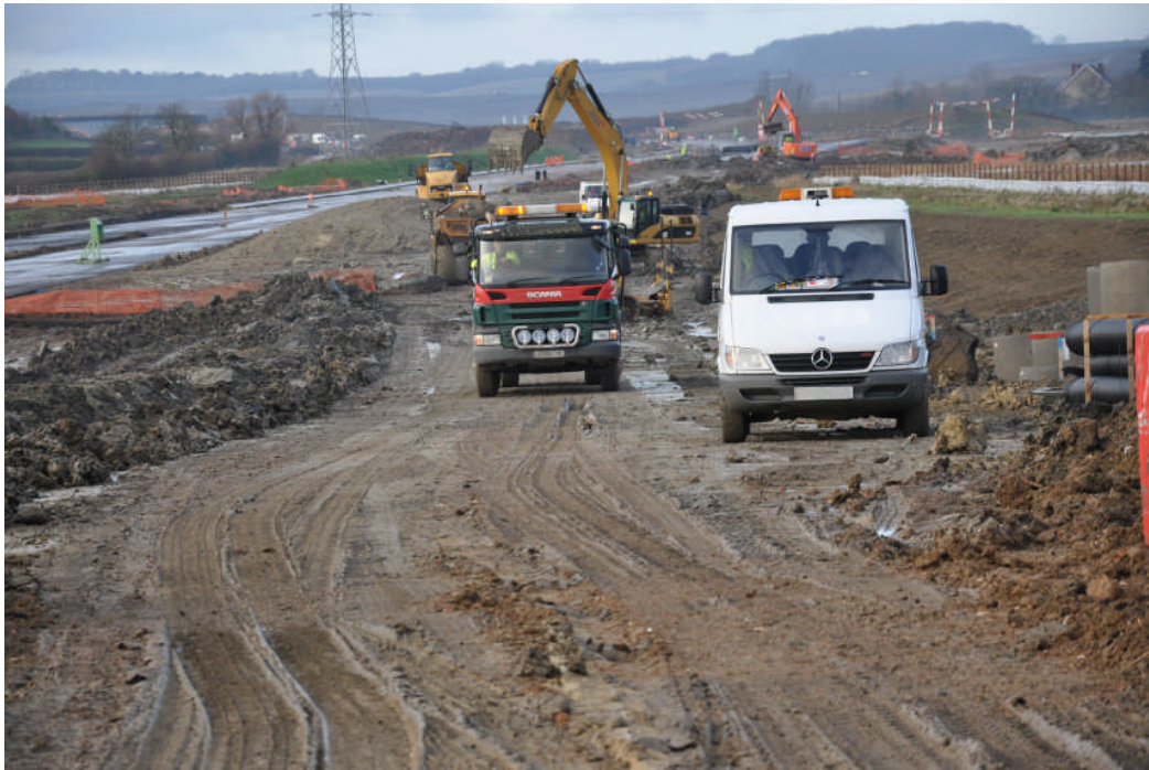
Figure 34 – Typical construction truck road used by 8x4 construction truck's to deliver aggregate.
