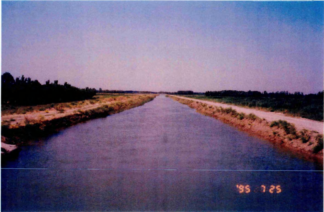
Figure 2-10. An unlined main canal in the Moghan scheme.
