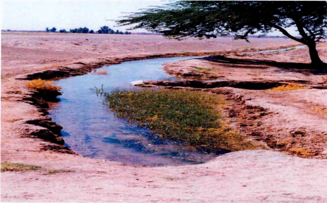
Figure 3-1. Poor condition of a tertiary canal in the Dez scheme.
