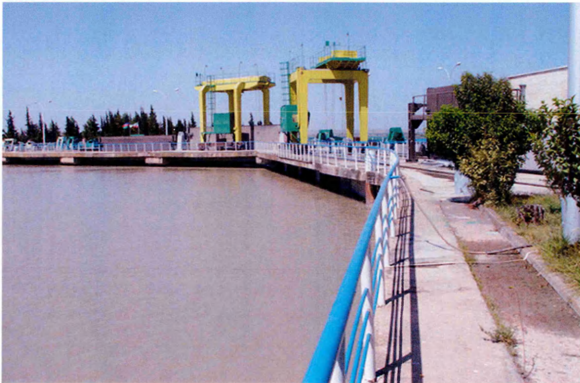
Figure 2-7. The Milo-Moghan Diversion Dam and Reservoir
