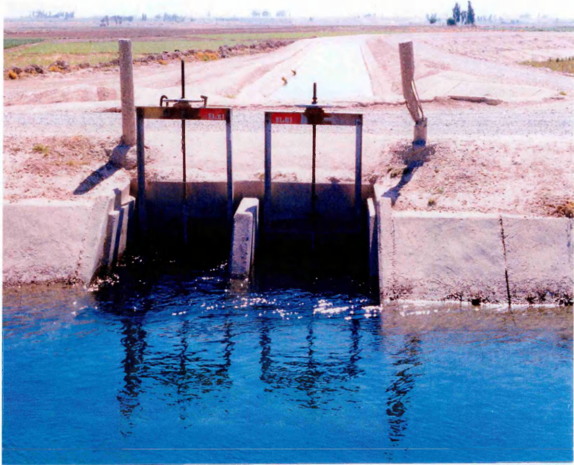
Figure 2-5. Regulator off the main canal in the Dez scheme.
