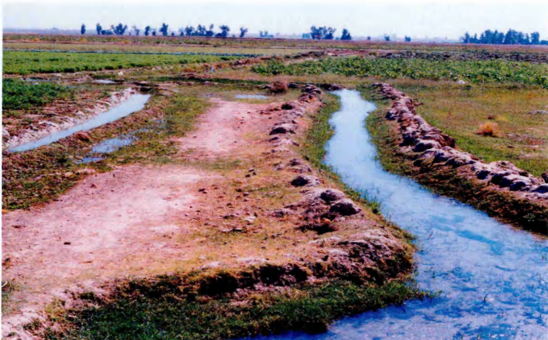
Figure 3-2. Seepage from a tertiary canal in the Dez scheme
