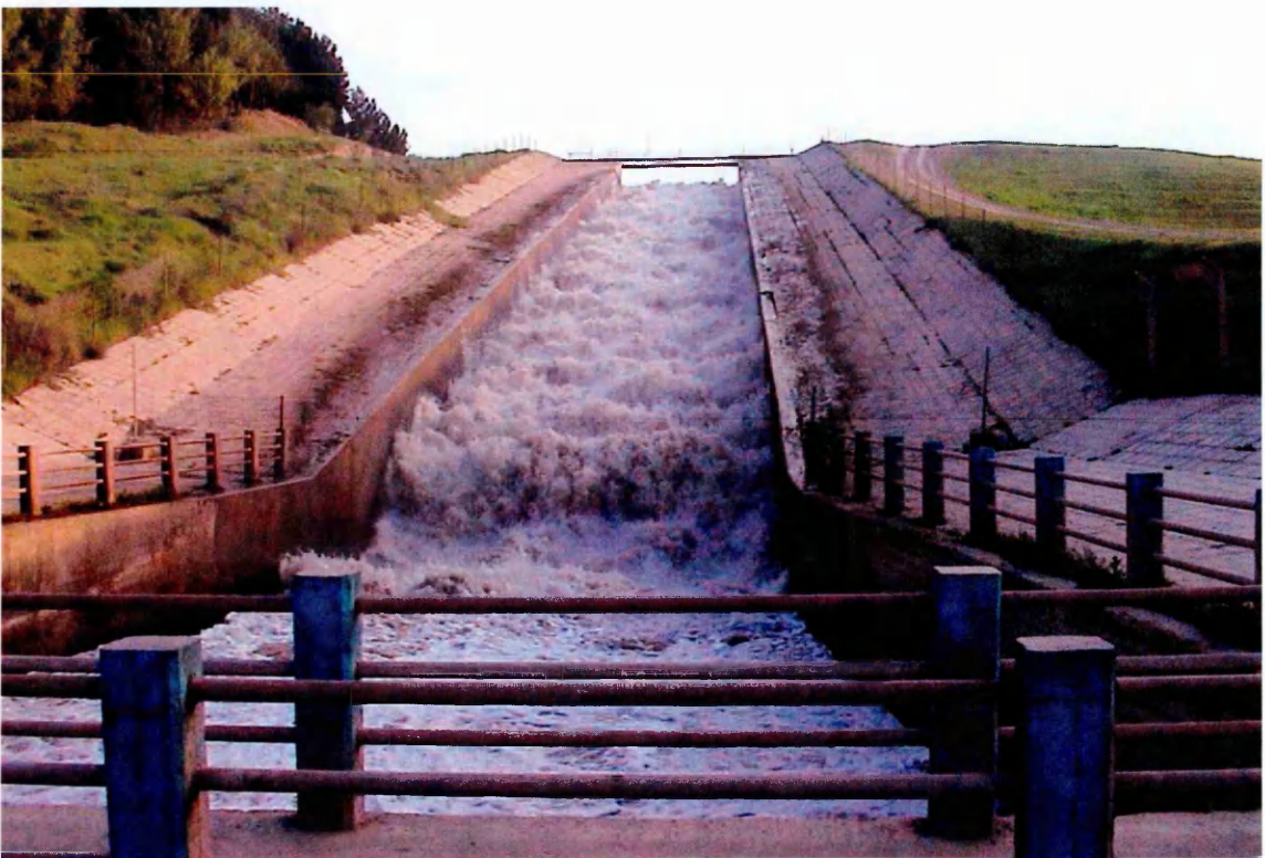
Figure 2-9. A chute in the main canal in the Moghan scheme.
