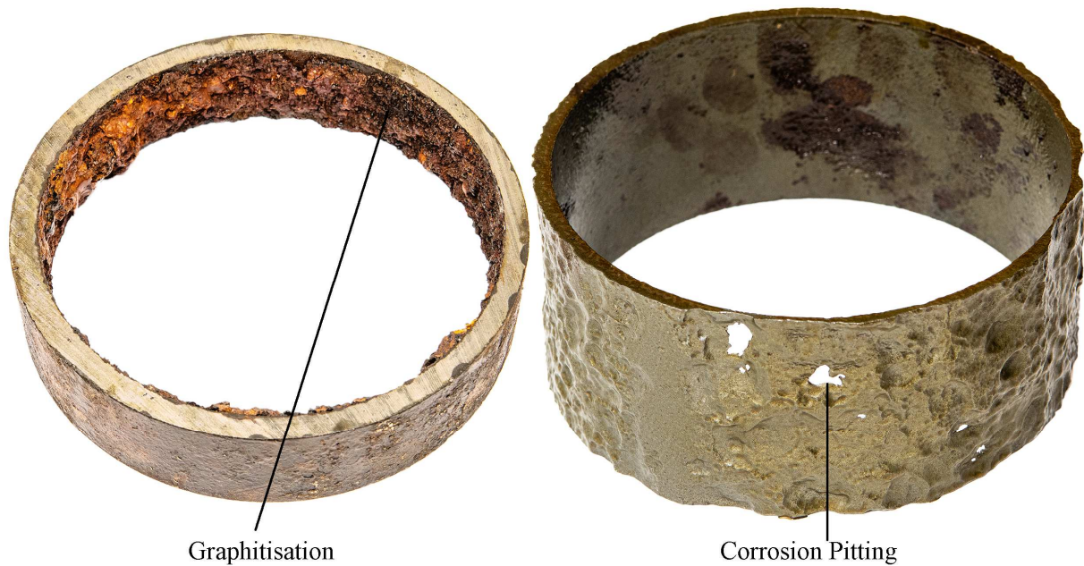
Figure 6. Cast iron pipe corrosion and chemical degradation.
