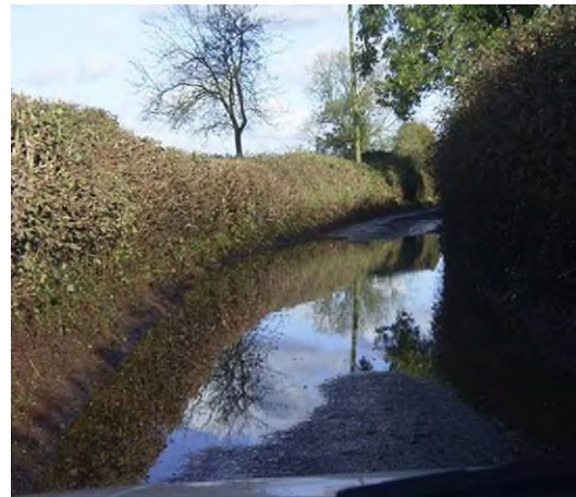
Local road flooding
