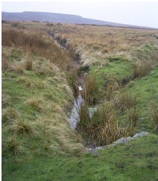
Drainage of moorland
