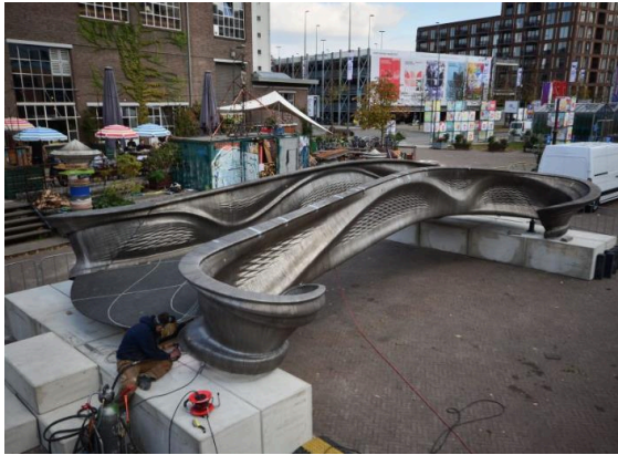
Figure 1. MX3D bridge (Liwanag, 2020).
