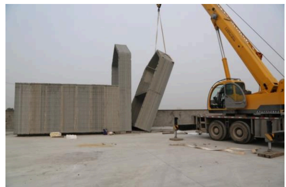
Figure 4. Assembly process of houses printed by WinSun (Deckert, 2015)
