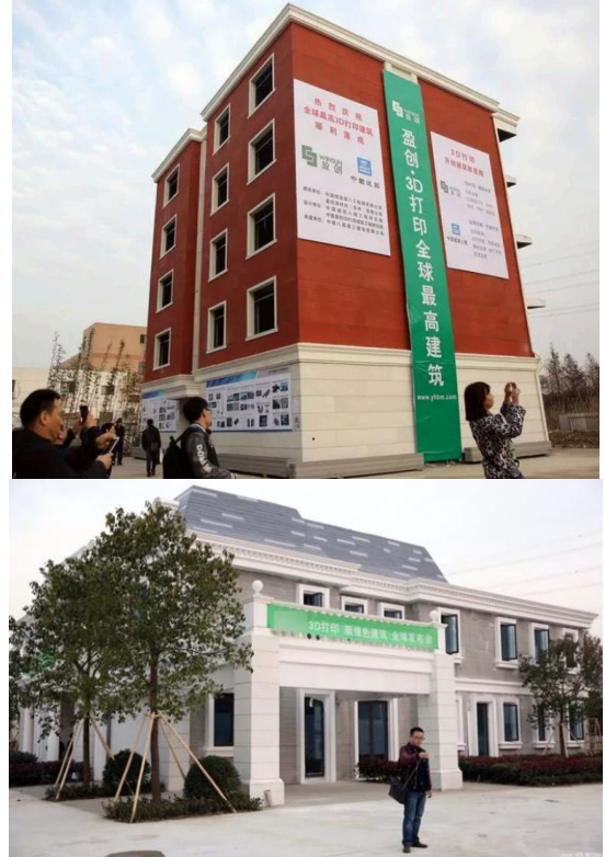
Figure 3. 3D printed buildings by WinSun (Starr, 2015).
