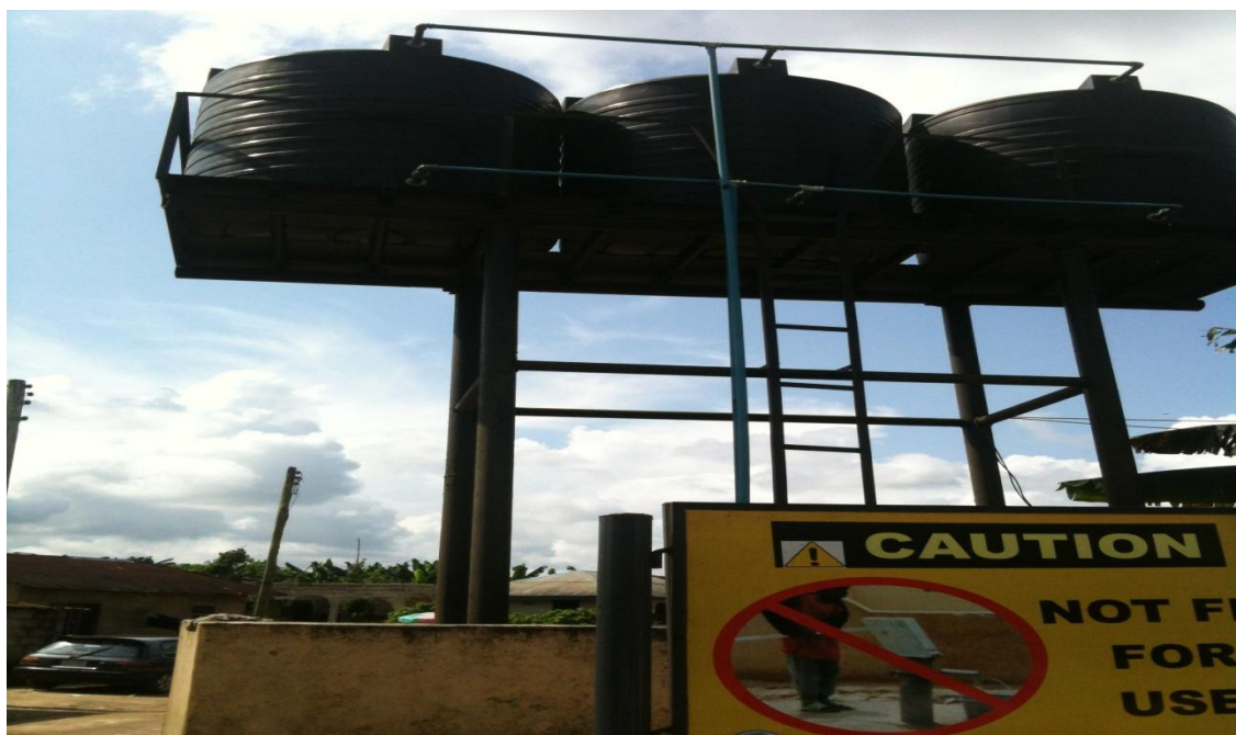
Figure 2-3. Water borehole in Ogale labelled as not fit for use.
