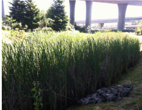
Figure 4-6. Bioswale at San Francisco International Airport Exit Ramp (Leda, 2012).
