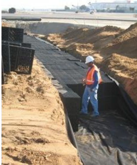
Figure 4-7. Bioswale installation at Los Angeles International Airport (Ecorainwater Solutions, 2023).
