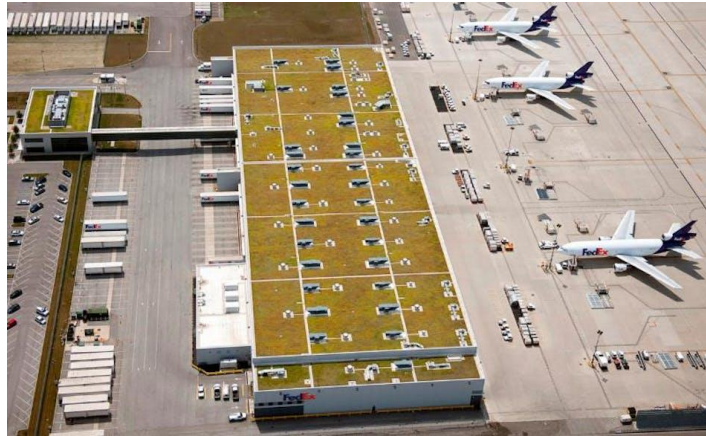
Figure 4-4. FedEx Main Sort Building, Chicago O'Hare Airport (Aviation Pros, 2016).
