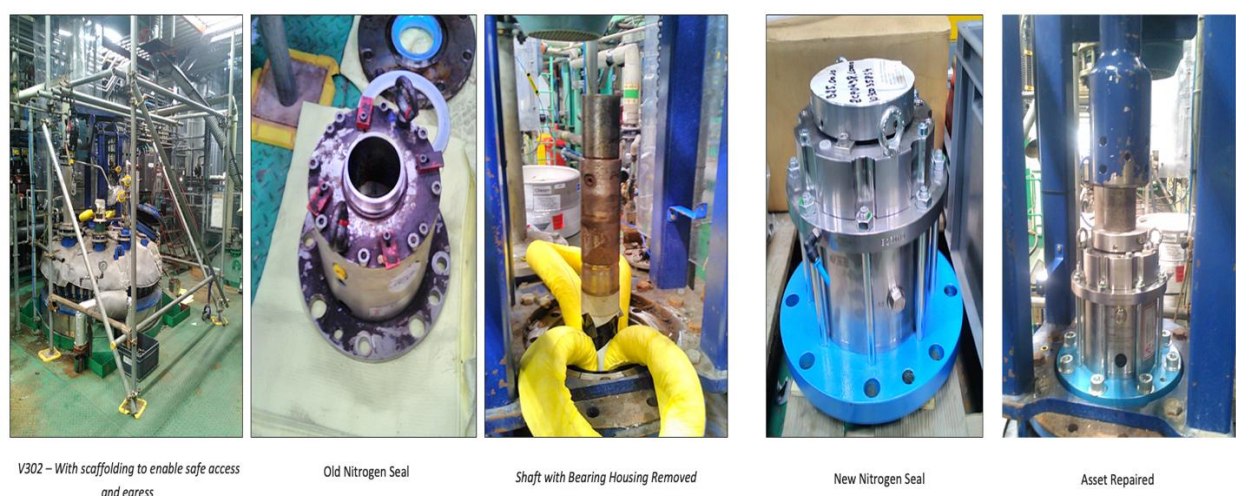
Figure 31 Pictorial storyboard of V302 repair
