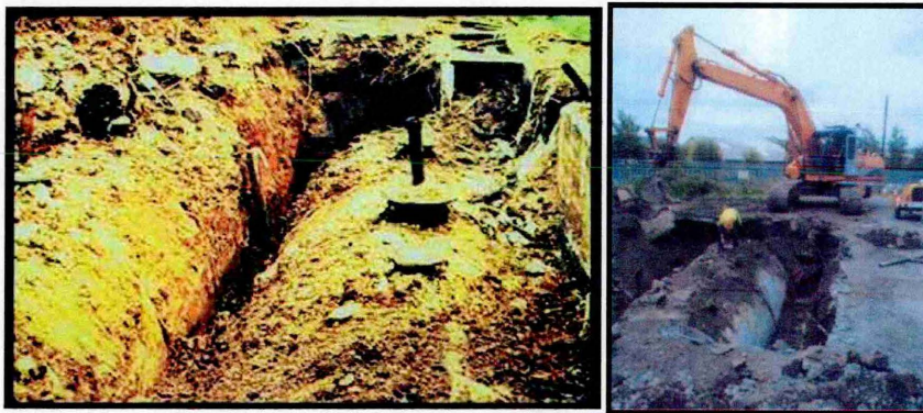
Fig. 1.1 Excavation of corroded & leaking UST
