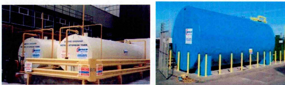
Fig. 1.2 Modern (post-2004) above-ground fuel storage tanks
