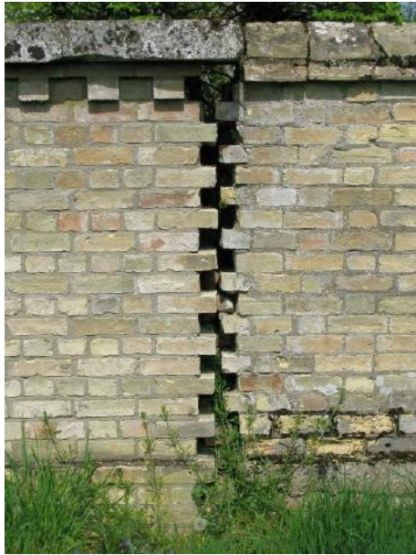
Figure 1 The effects of severe clay-related movement on brickwork.(Wimpole, Cambs. S. Hallett)
