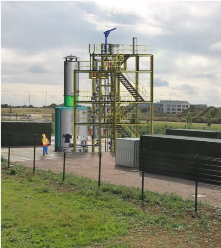
Figure 7: Test site at Cranfield University with rendering of 1 MW th CHG pilot plant to start operation in 2022 (BEIS “HyPER” project).
