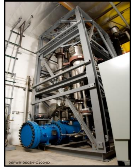
Figure 4: Original CHG pilot plant (0.071 MW th ).
