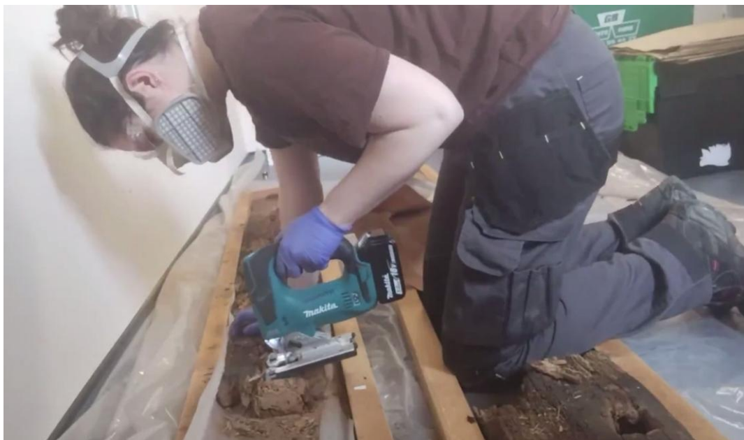
Figure 36: The author cutting the plank with a jigsaw on the storeroom floor (phone on stand).
