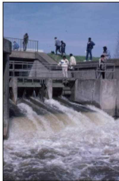
Figure 2.6 Neyrpic gate at Denver Sluice. Controlled rate of discharge (Photo T.M. Hess)
