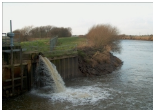
Figure 2.8 Beckingham Pumping Station
