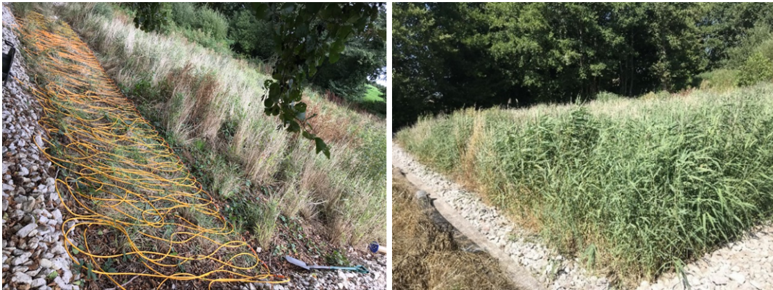
Figure 2-4 Recently refurbished HSFCW
