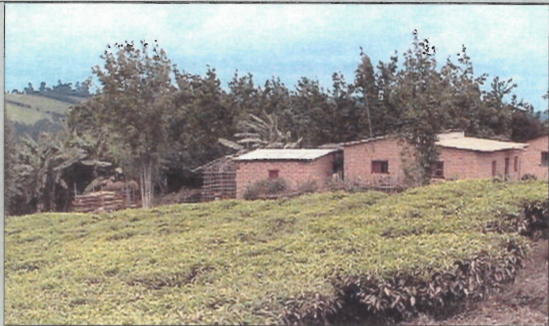
PLATE 4.4: Iron roofed buildings in rural areas indicate a wealthy household
