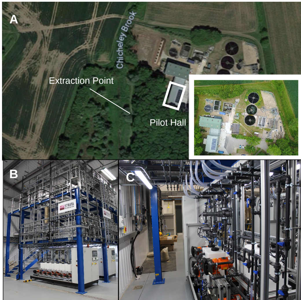
Figure 3: A. The location of the National Research Facility for Water and Wastewater Treatment (NRF-WWT) at Cranfield University, coupled with the designated abstraction point along Chicheley Brook. This specific point was utilized for sourcing water in the pilot-scale experiments. B. A detailed depiction of the near-real scale drinking water treatment rig. This photo showcases the rig's design and layout to mimic real-world water treatment processes. C. Underside of the drinking water treatment rig's structural and functional components.
