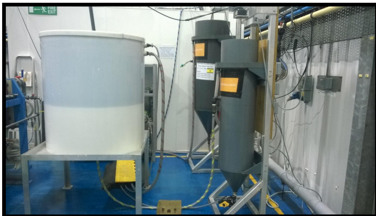
Figure 3.1. Picture of pilot-plant showing the set-up of the primary and final sedimentation tanks (grey PVC tanks) and the mixed liquor tank (white PVC tank).
