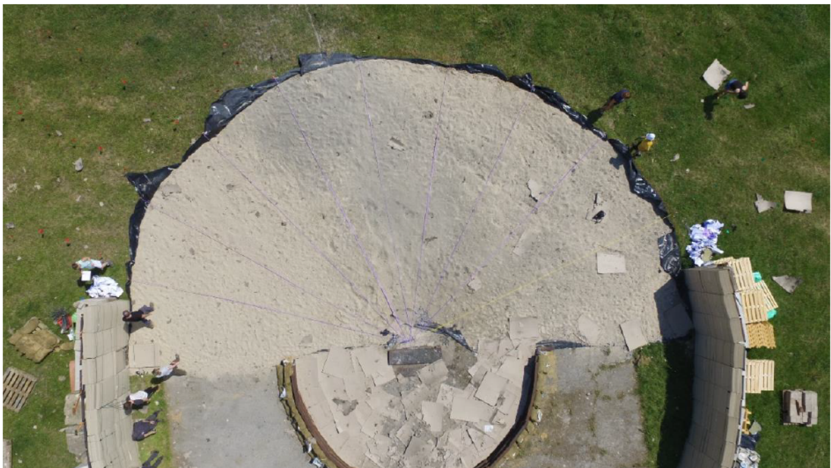
Figure 6. Aerial picture after detonation 1.
