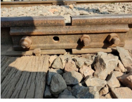
Fig. 4. Broken fishplate.
