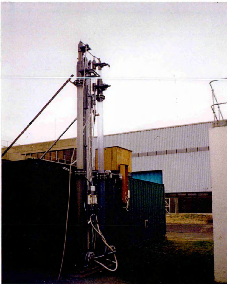
Plate 2. Ozonation Columns Mounted on Pilot Plant Clarifier.
