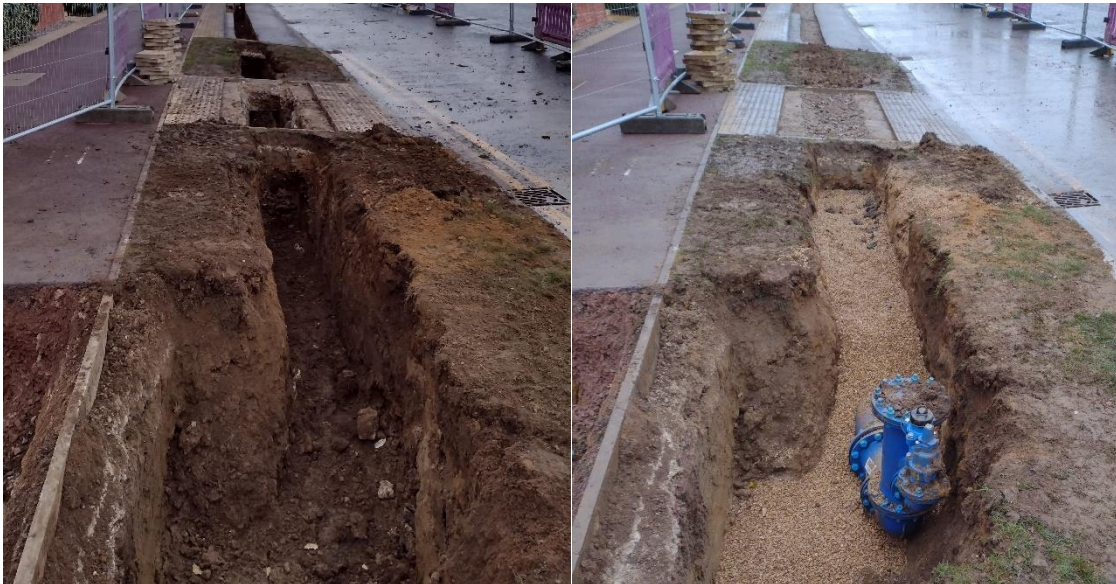
Figure 7-2 Pipe installations showing the removal of local soil conditions, and installation of pipe bedding and backfill (Photos taken by author).
