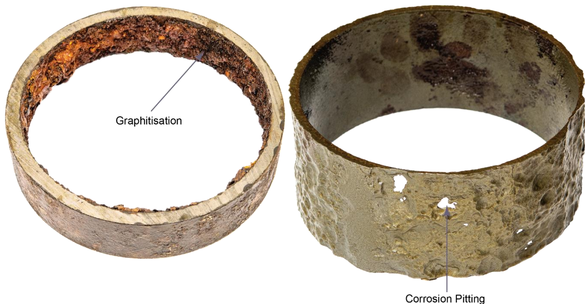
Figure 2-6 Cast iron pipe corrosion and chemical degradation.
