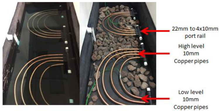
Figure 128: Eight 10 mm copper pipes on the basin with the 10 degree angle
